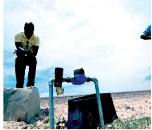
Water meter, Ompumbu settlement, Oshakati
