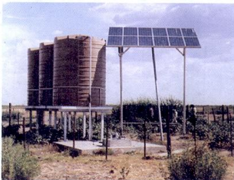
Solar water pump at Onandjendje Project.
